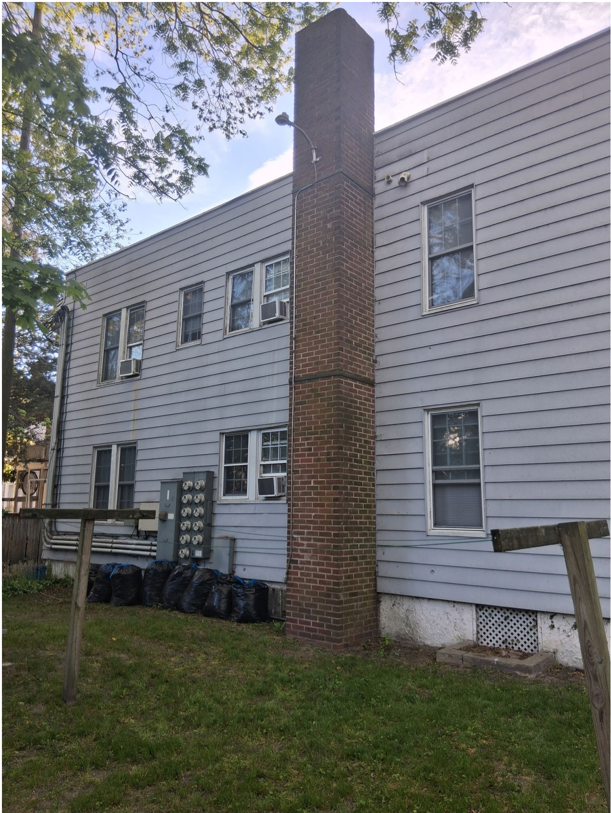
3 – Back Side of Building
