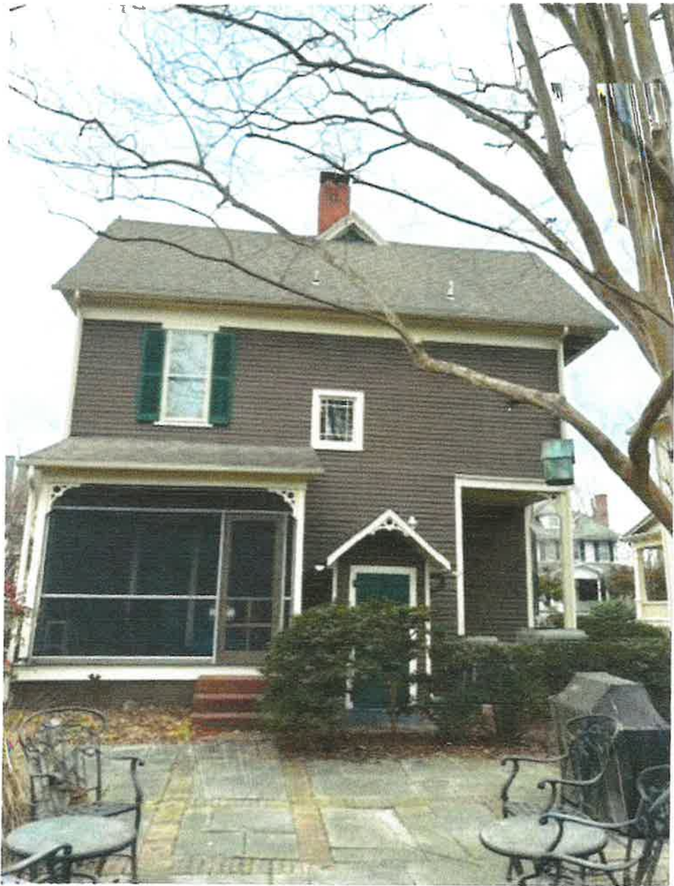
Rear of property at 104 Elizabeth
