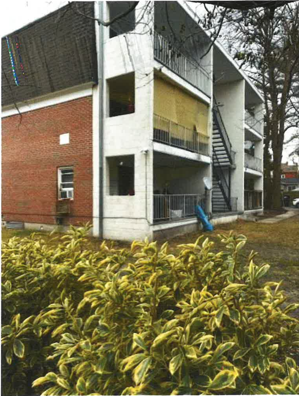
Rear of apartment building immediately adjacent at 108 - Elizabeth Street
