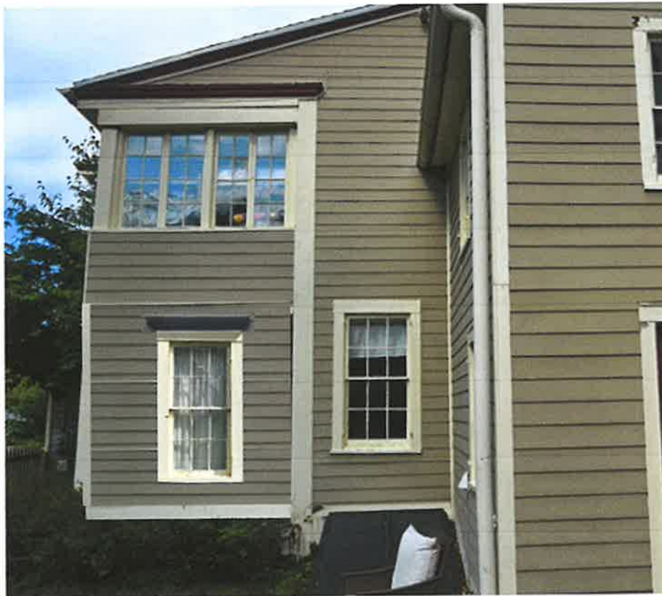
After – Side Porch from Back of House
