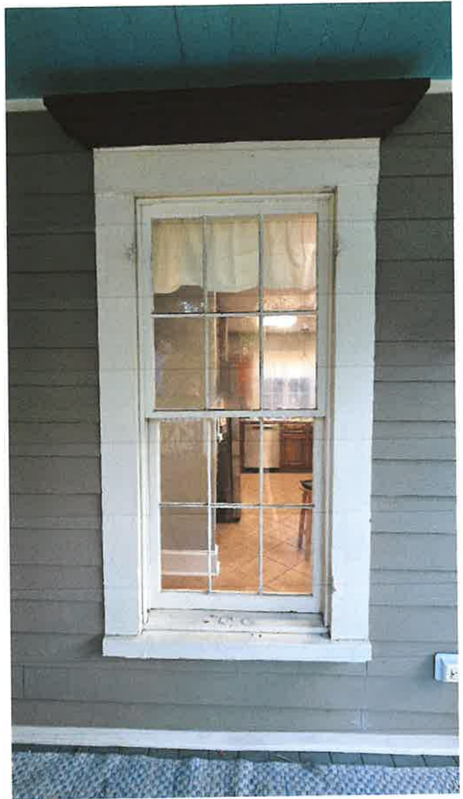
Window on exist Porch. Single Pane, 6 over 6 Wooden windows. Enclosed porch will include 3 of these style windows and trim with approximate dimensions of 32" x 72"
