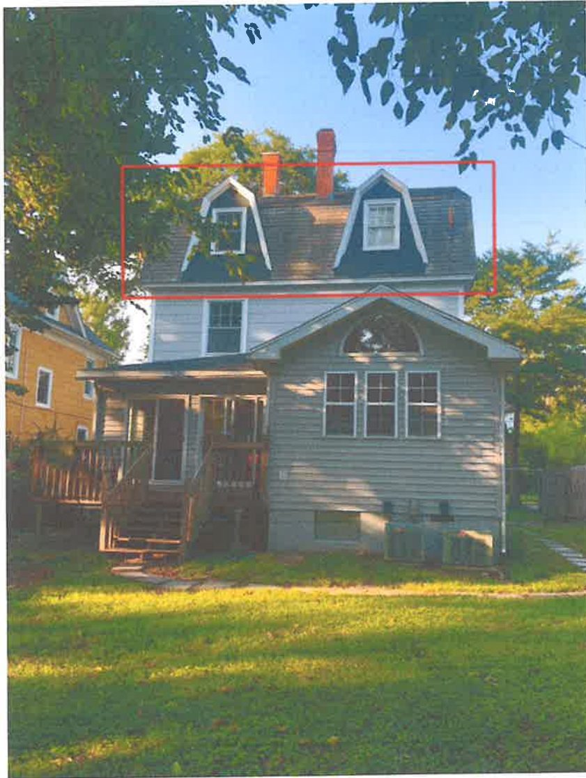
Figure 1. Rear of 116 Elizabeth St, showing portion of roof (outlined in red) where asbestos shingles are to be replaced with asphalt shingles.
