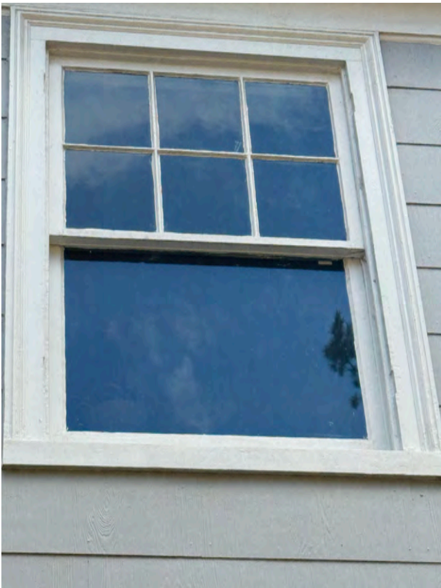
RIGHT SIDE OF HOME, SECOND FLOOR
