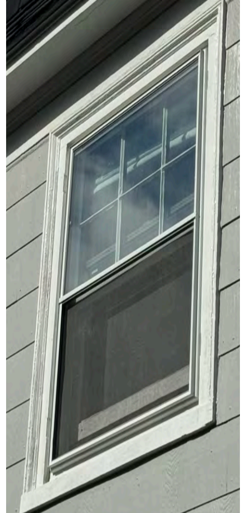
LEFT SIDE OF HOME, 2ND FLOOR
