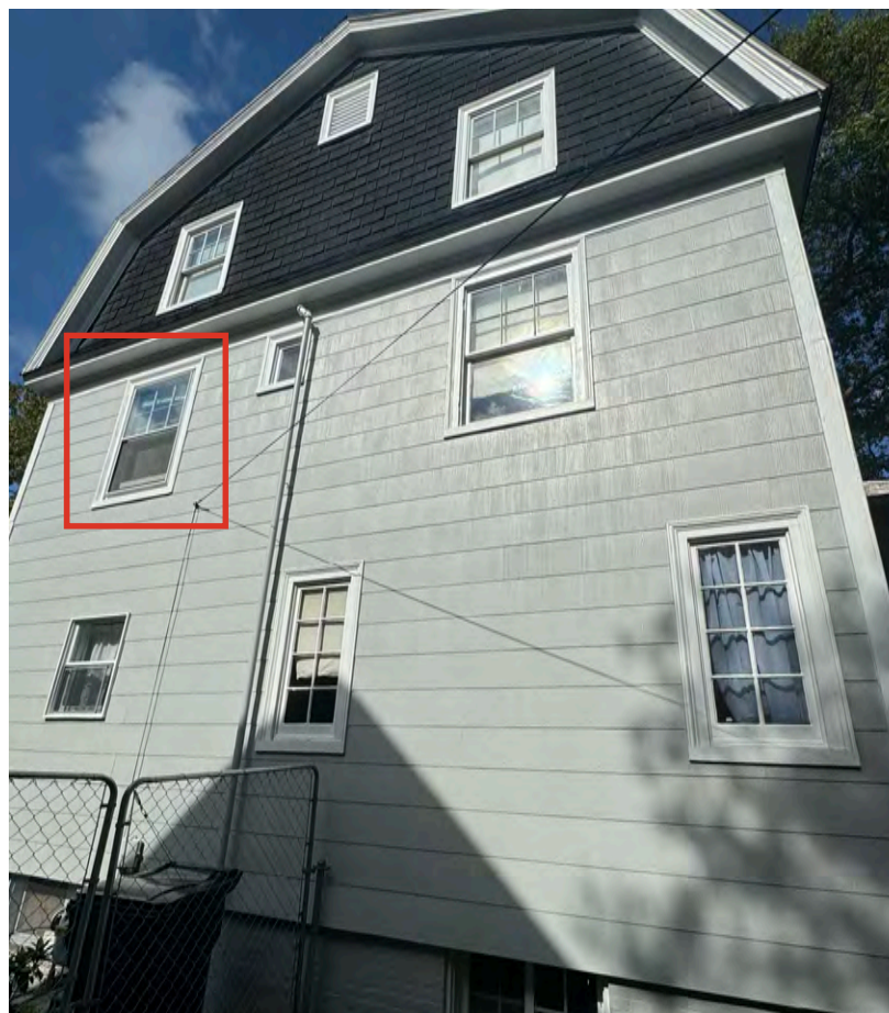
LEFT SIDE OF HOME 1 WINDOW PROPOSED FOR REPLACEMENT MARKED IN RED
