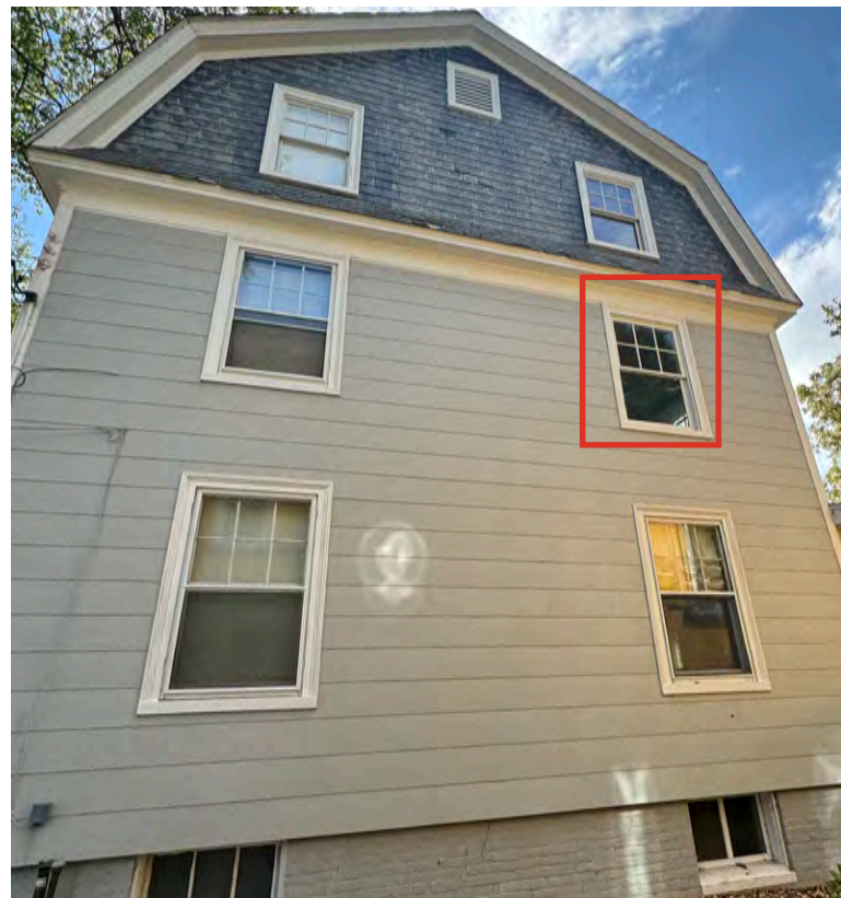
RIGHT SIDE OF HOME 1 WINDOW PROPOSED FOR REPLACEMENT MARKED IN RED
