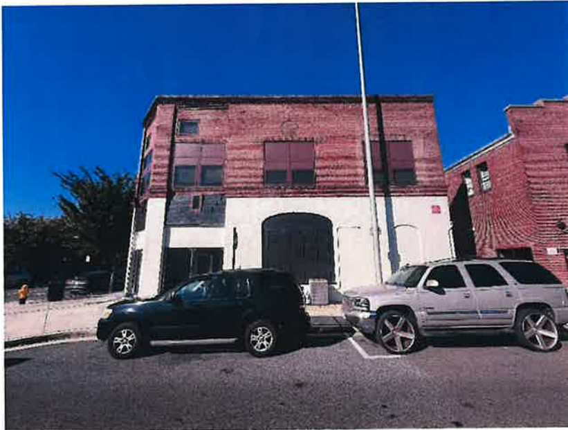
Structures Opposite West Façade.
