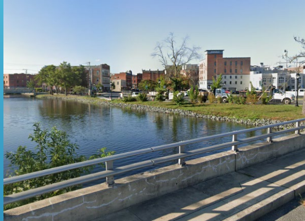
Shoreline Restoration: Such as Mill Street Shoreline Restoration.
