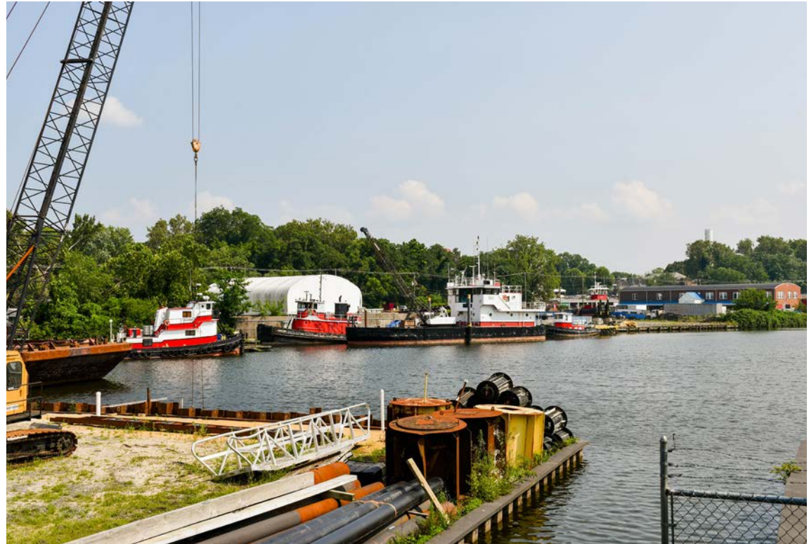
North Prong Wicomico River, working waterfront. Courtesy City of Salisbury.
