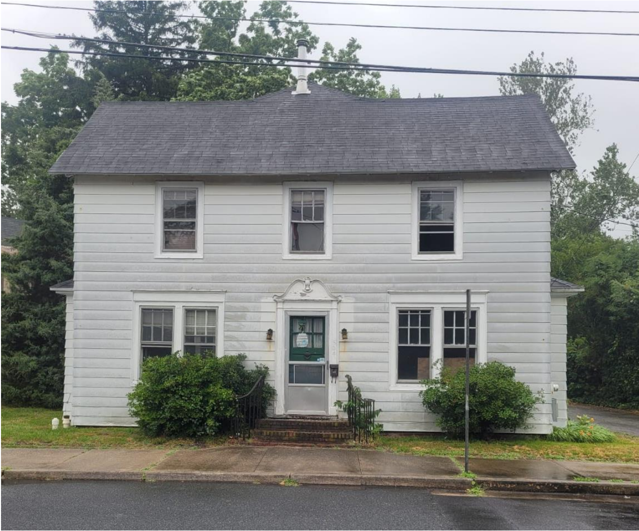
Neighboring property: 304 Poplar Hill Ave (Right)
