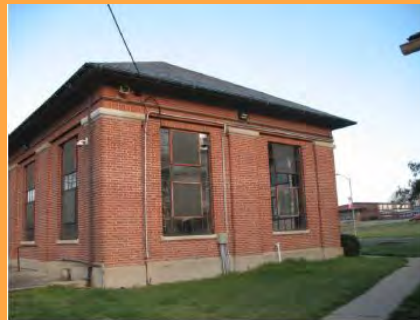
Photograph 2-1: Pump Building Looking from the East
