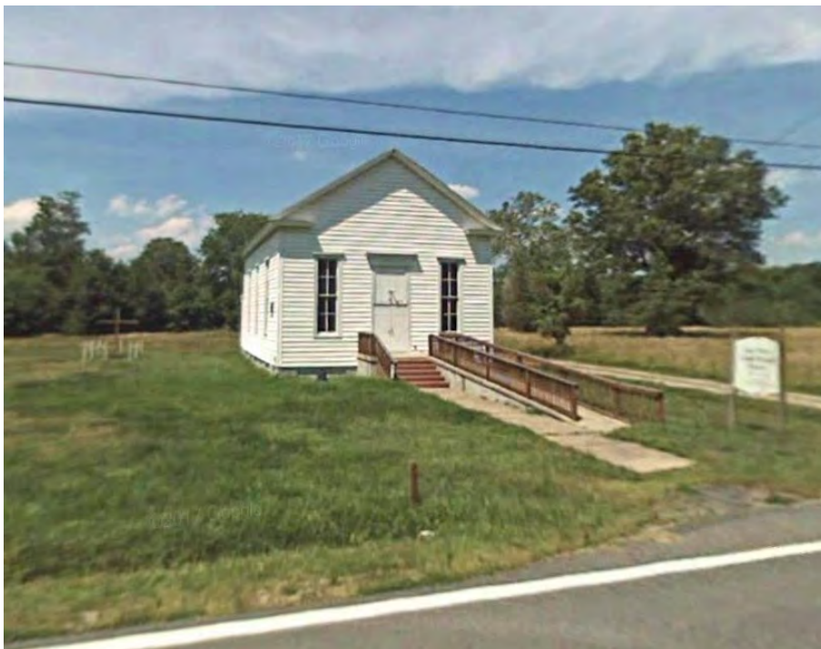
John Wesley Methodist Church Located on Capitola Road in Tyaskin. This church is at-risk to the 1% annual chance flood event.
