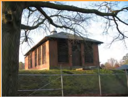
Photograph 2-3: Aerator Building Looking from the North
