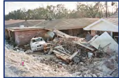
Canal levee breaches as a result of Hurricane Katrina in New Orleans in 2005. Note damages can be more extensive due to high velocity flood flows than if the levee was not there.
