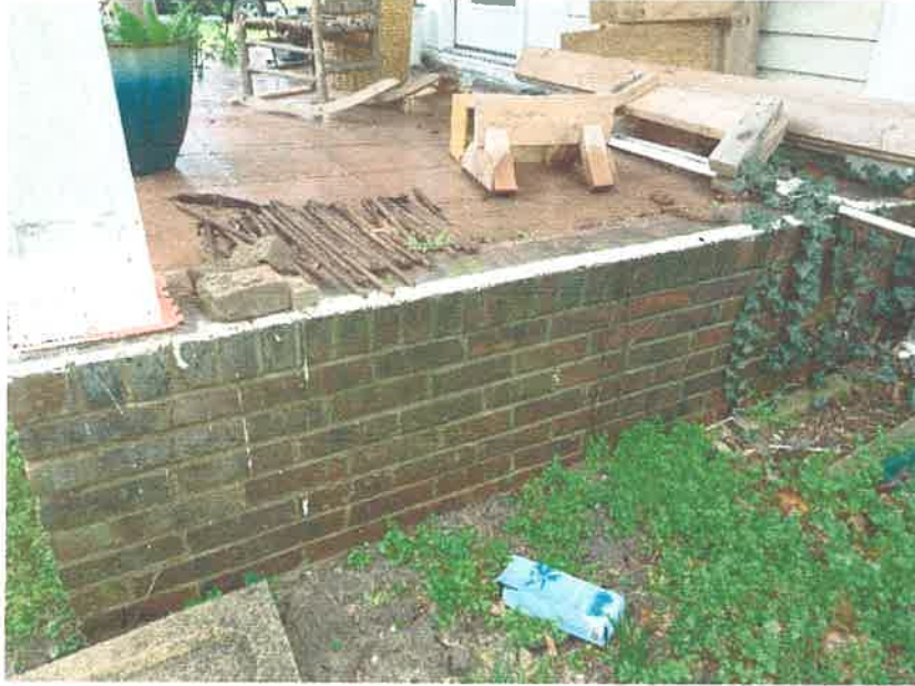
Rear view of foundation
