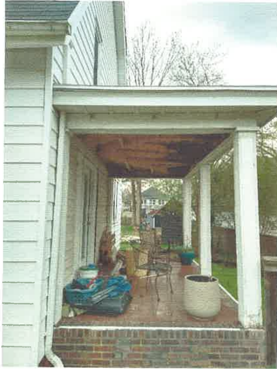
303 Middle Blvd close up of porch/sunroom from front yard
