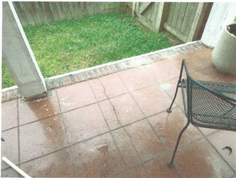
Poured concrete floor
