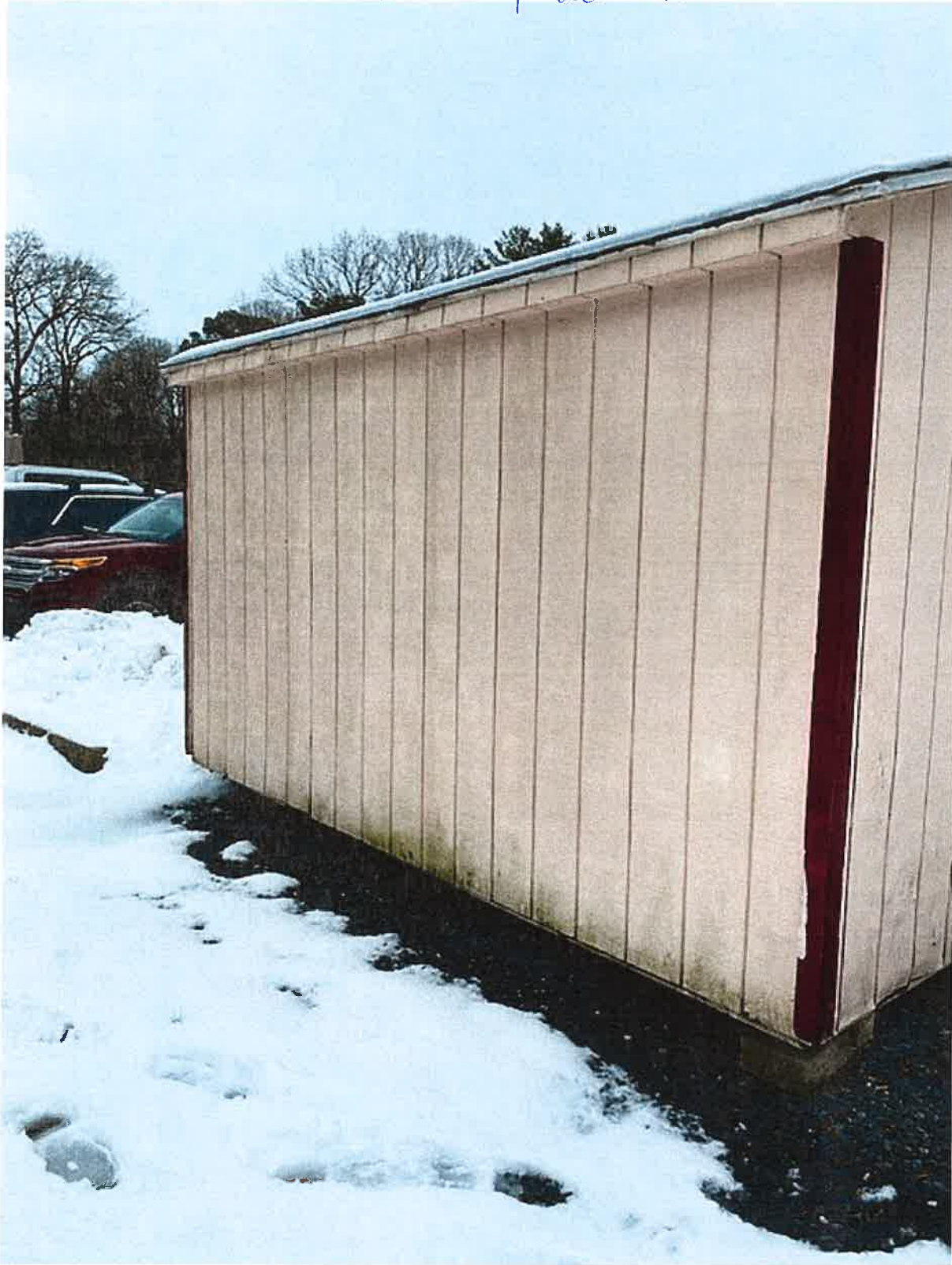
Left - Replacement shed
