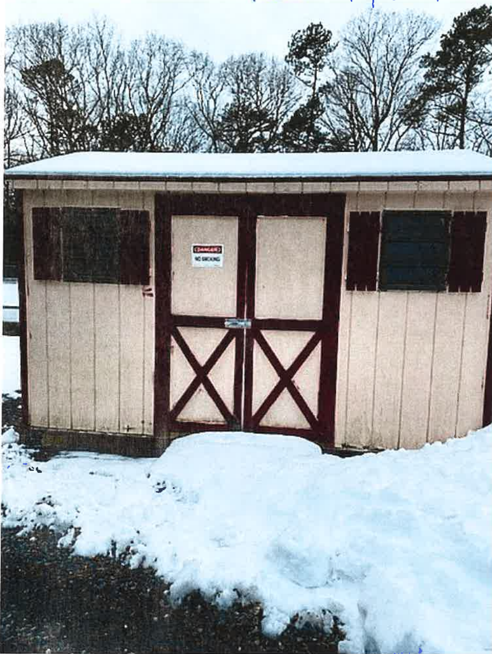
front - replacement shed
