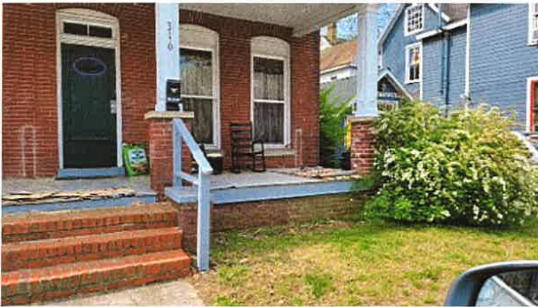
314 Maryland Front Porch
