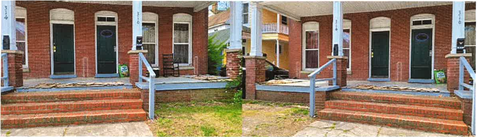
314 Maryland Front Porch
