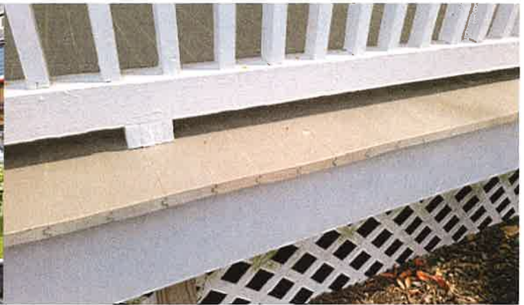
311 Maryland Front Porch
