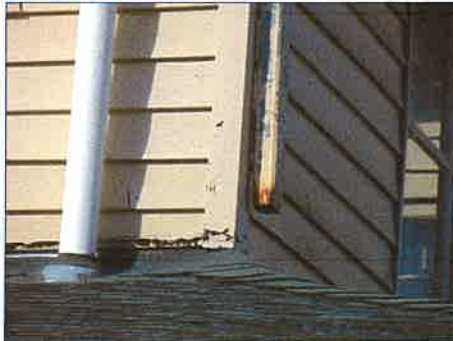
Elbow not installed.
