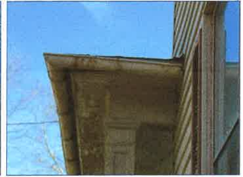
Gutters are not adequately secured to the roof.
