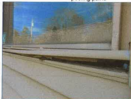
Vinyl trim not installed properly.
