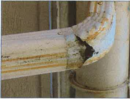
Gutters and downspouts are considerably rusted.
