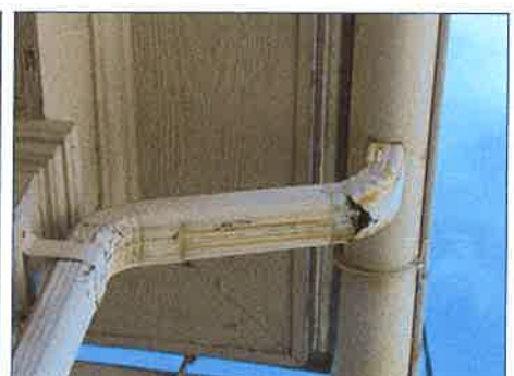
Gutters and downspouts are considerably rusted.
