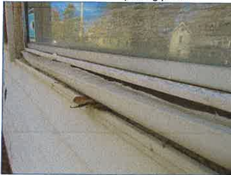
Vinyl trim not installed properly.
