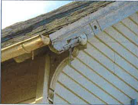
Bare wood and peeling paint.
