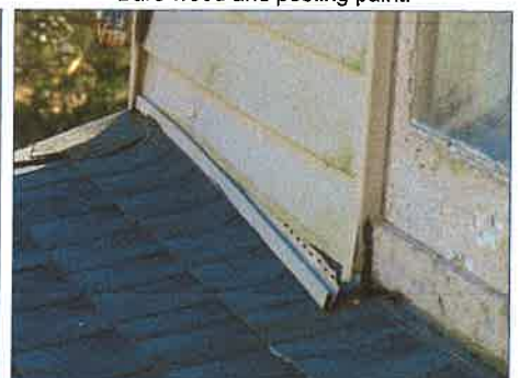
Vinyl trim not installed properly.
