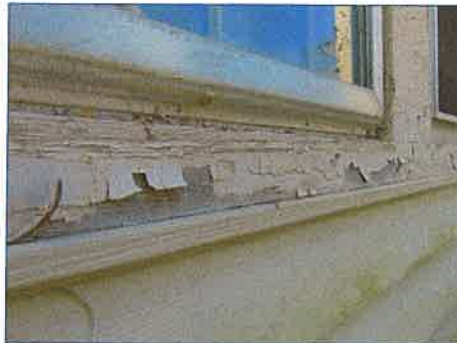
Bare wood and peeling paint.
