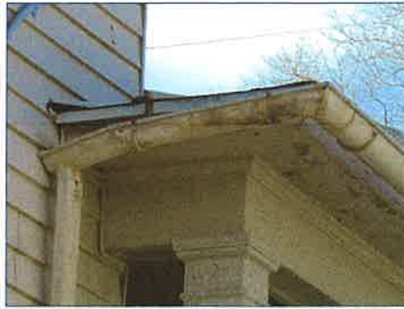
Gutters are not adequately secured to the roof.
