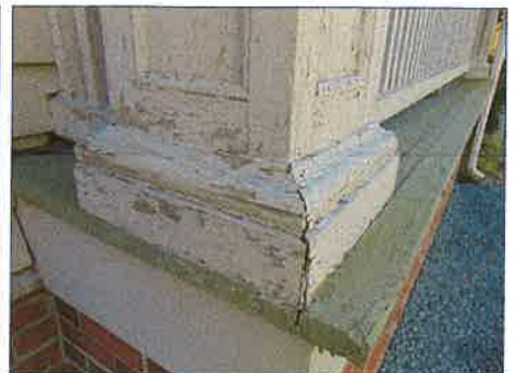
Bare wood and peeling paint.
