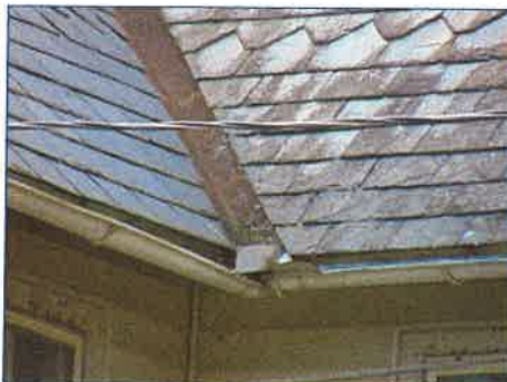
Damaged gutters.
