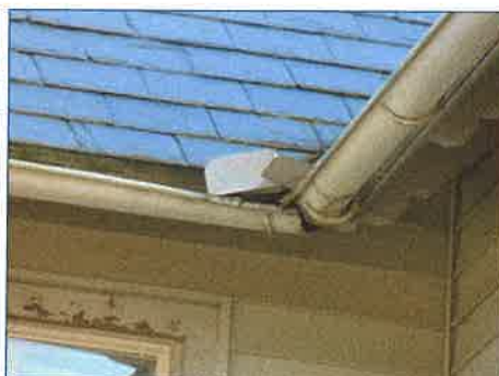
Damaged gutters.
