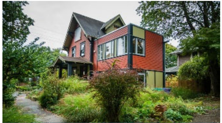
Example of an attached ADU in Portland, Oregon. Image from: https://www.portlandoregon.gov/hps/article/930137
