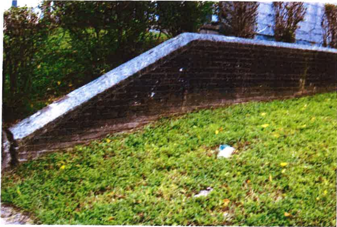
WEST SIDE OF THE ORIGINAL RETAINING WALL
