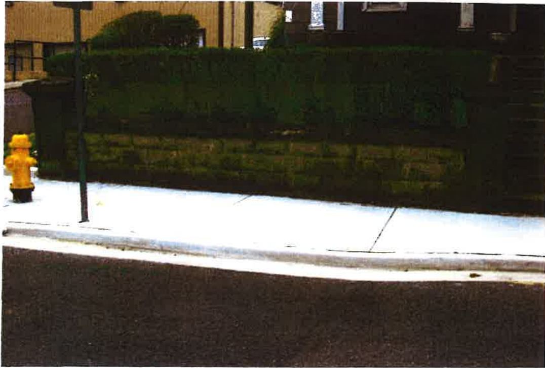
EAST SECTION OF THE RETAINING WALL
