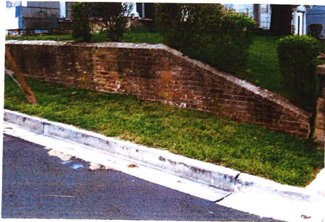
EAST SIDE OF THE ORIGINAL RETAINING WALL
