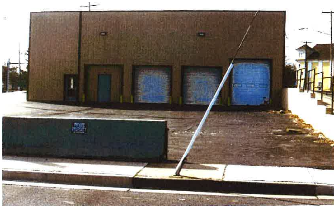
EAST SIDE PROPERTY ADJOINING 312 E. WILLIAM ST.
