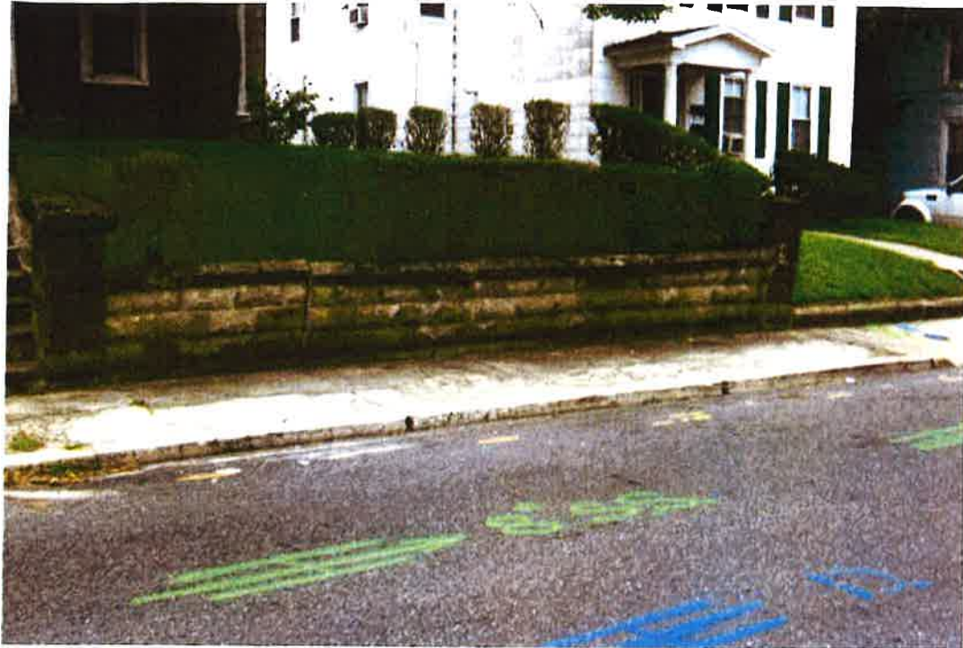
WEST SECTION OF THE RETAINING WALL
