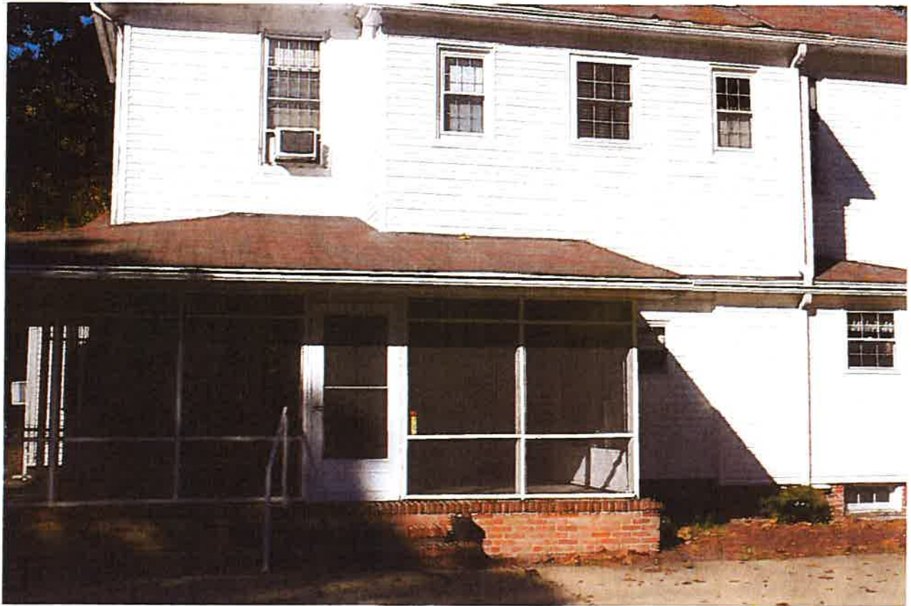
PHOTO - BACK ELEVATION 407 Camden Ave Salisbury, MD
