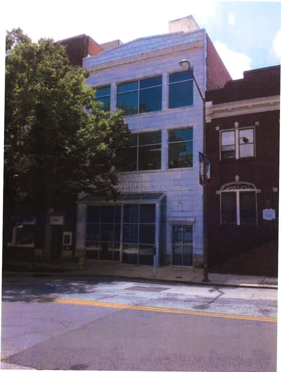
128 E. Main St Close up
