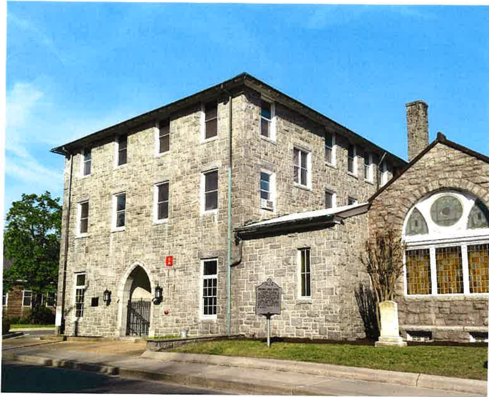
Looking Northeast from North Division Street
