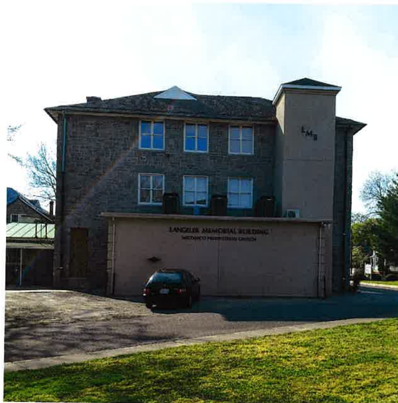
Back of 225 North Division Street Annex
