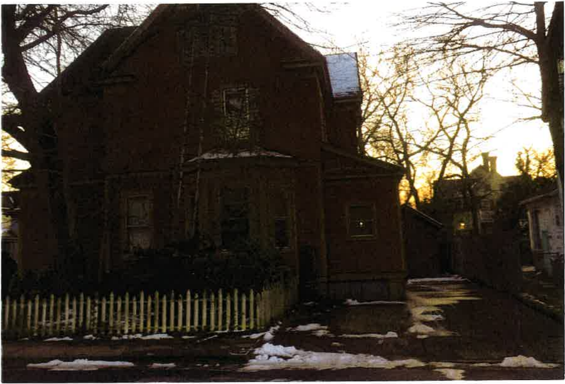
NEIGHBOR'S HOUSE EAST NORTH FACE
