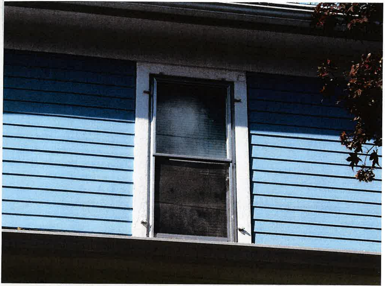
2 nd floor front Right window
