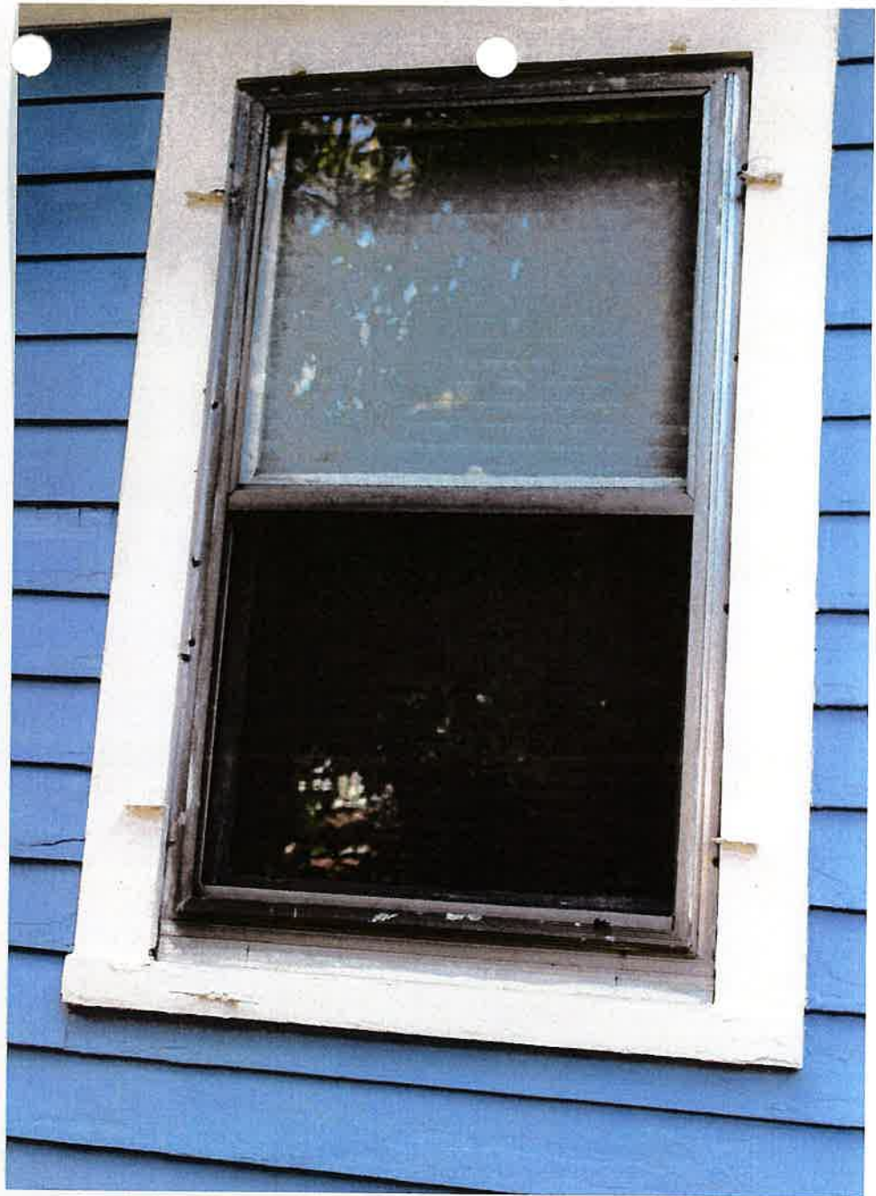
Back 11 1st floor window to the left
