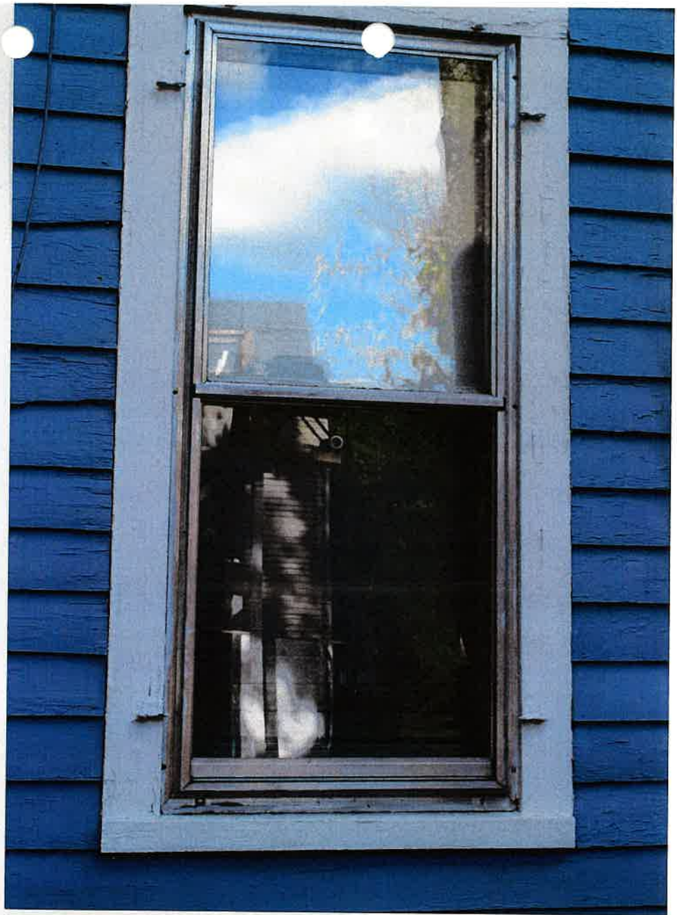
L - first floor 1st window
