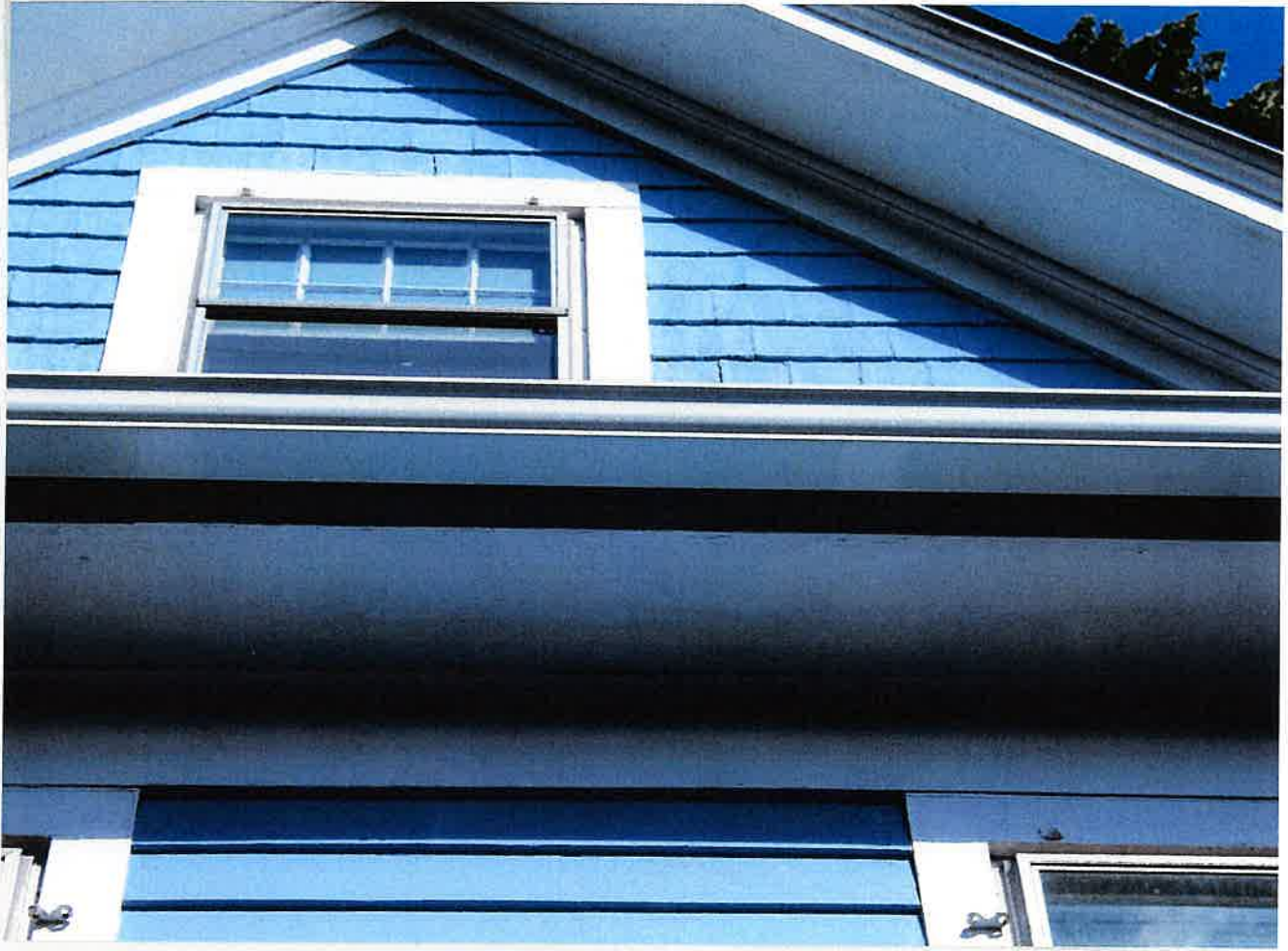
L-side attic window
