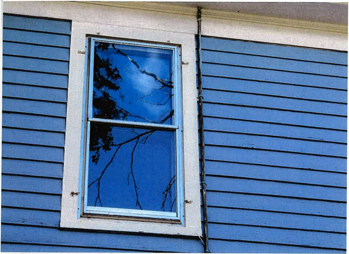
R-side 2 nd floor last window
