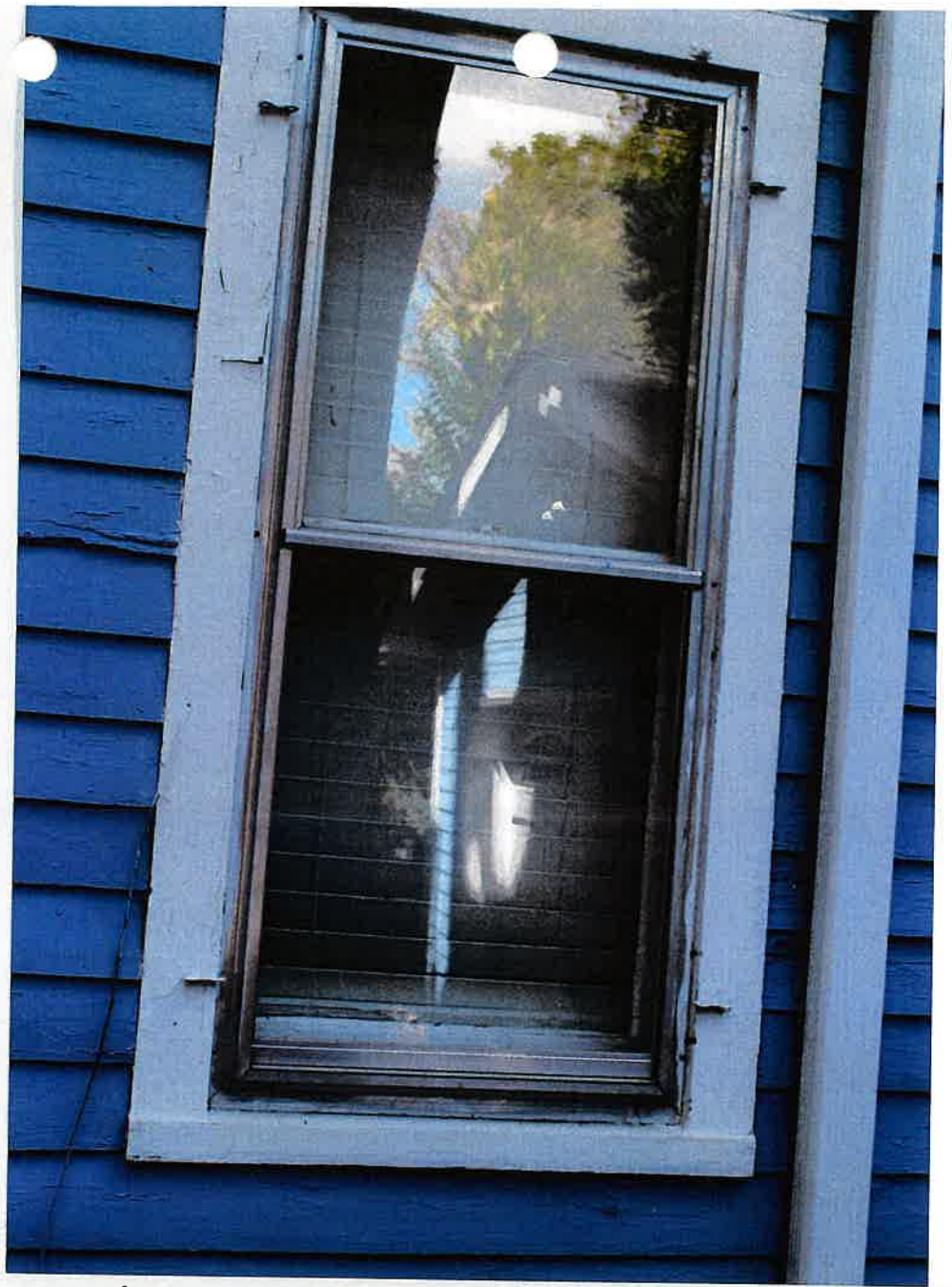
R-side first floor far window
