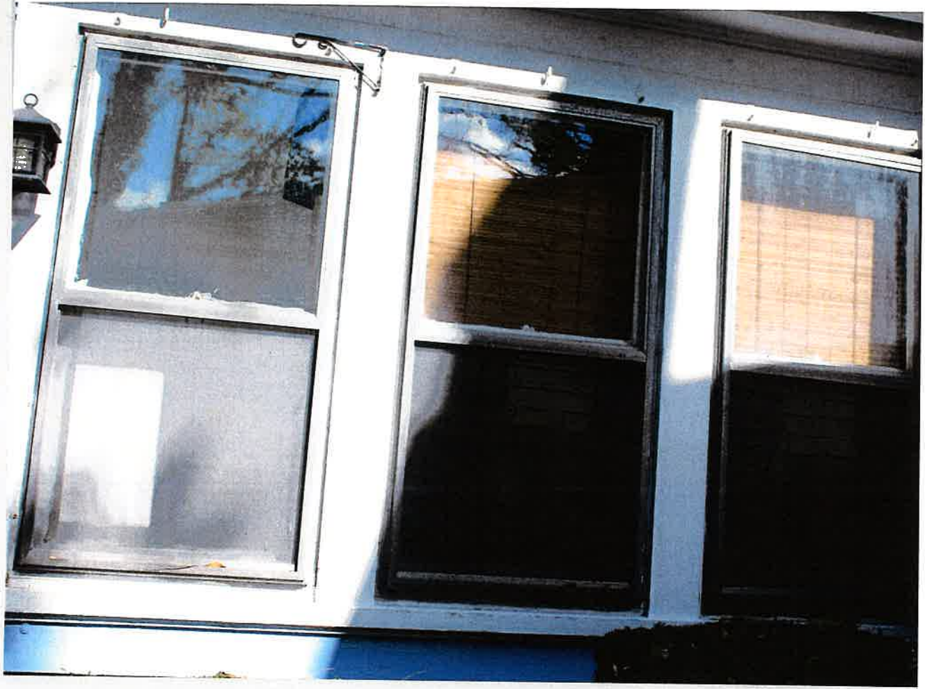
L-side first floor Back Windows
