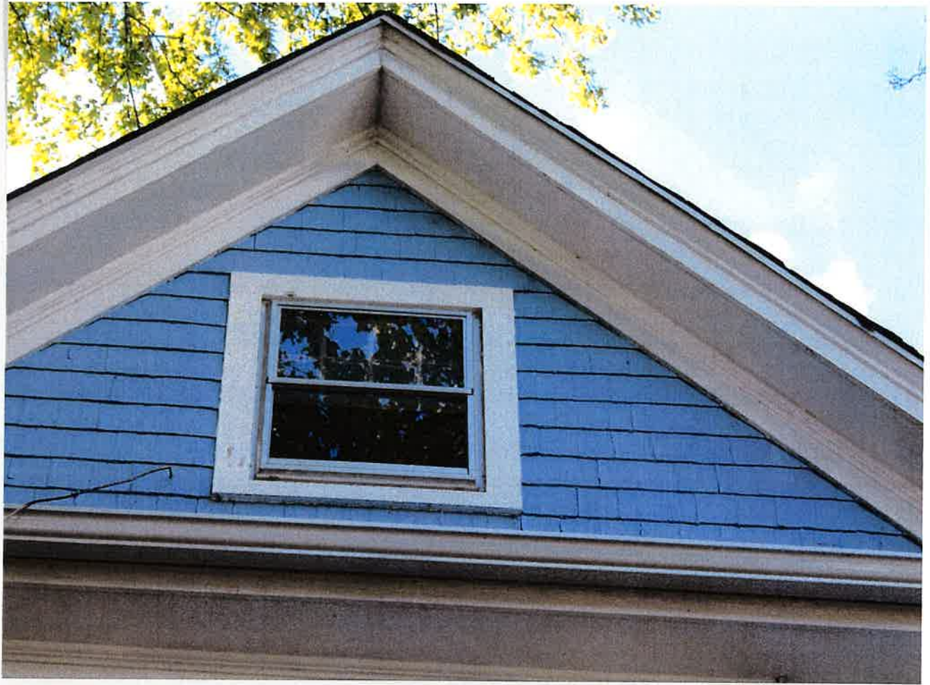
R-side attic window
