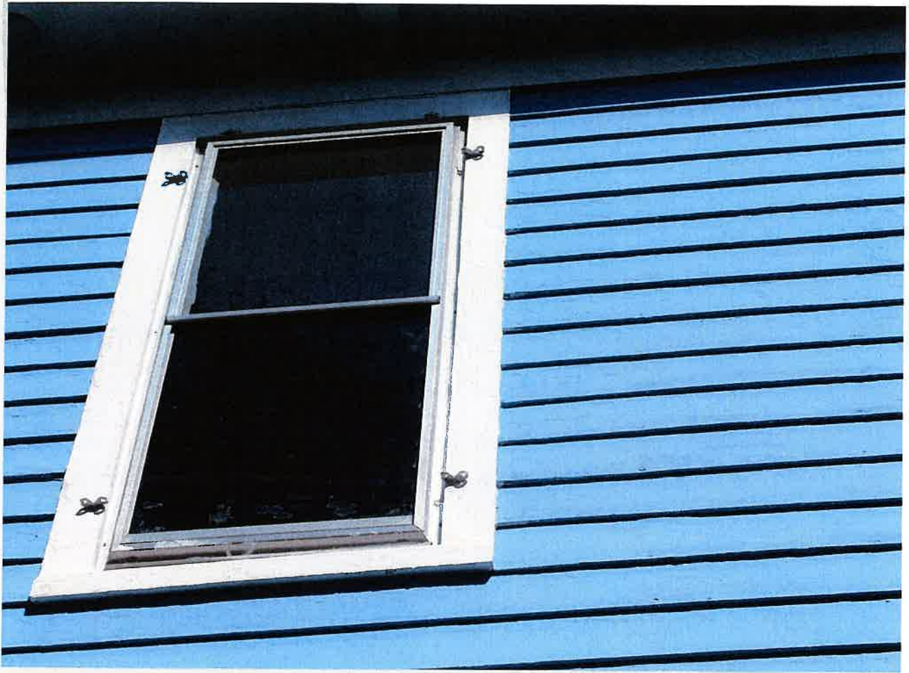
L-side 2 nd floor 3 rd window
