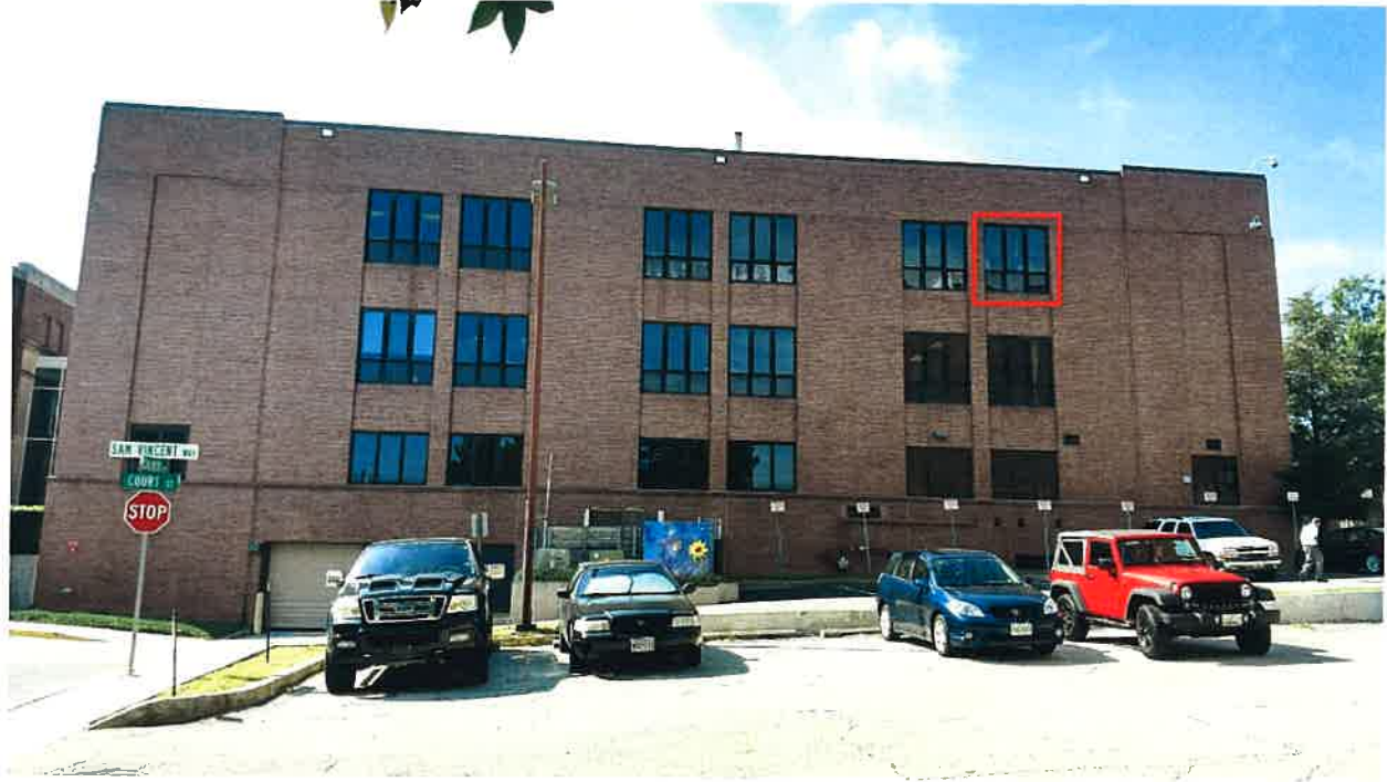
East Façade (Window Highlights in red will be replaced)
