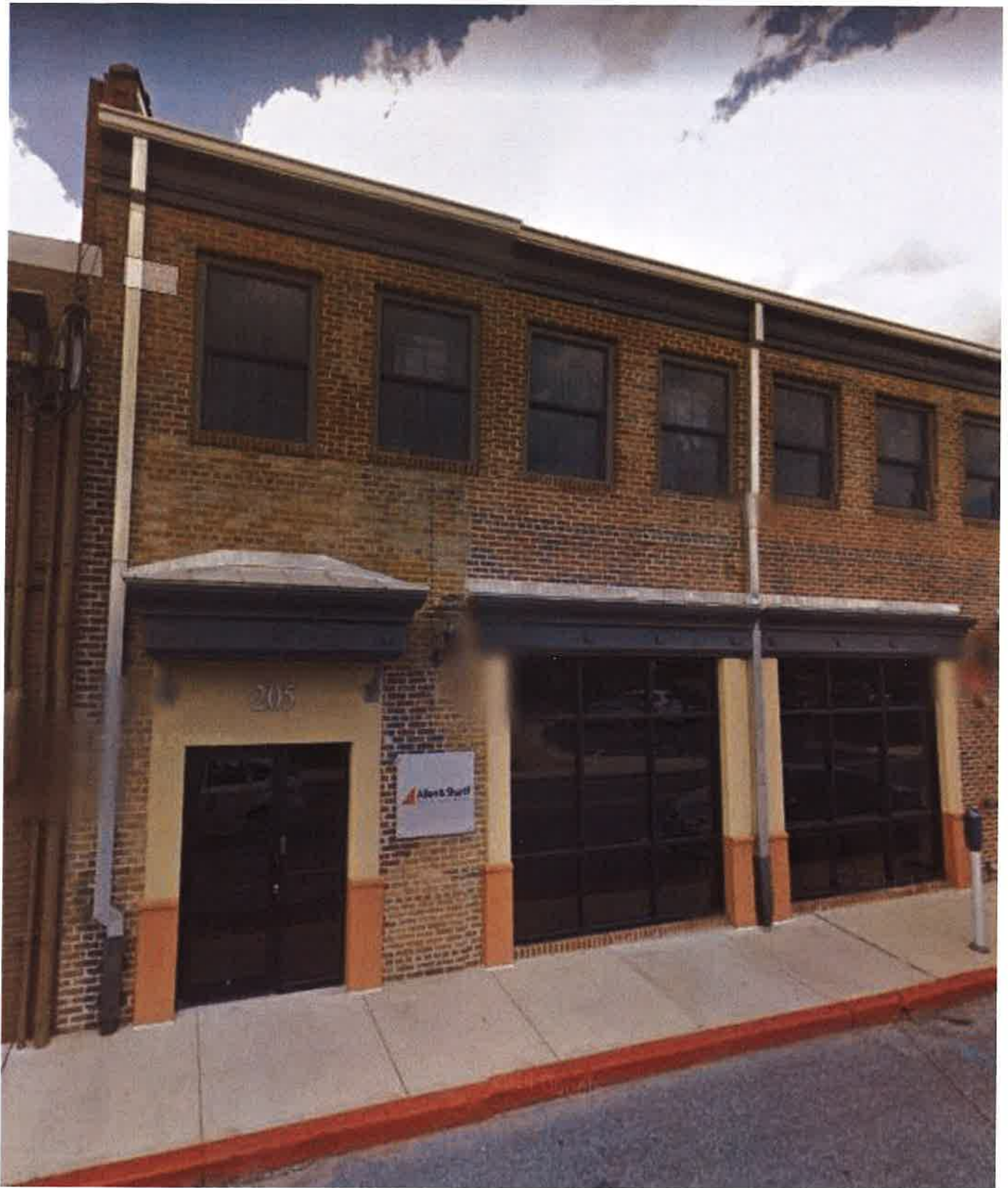
Neighbor to the Northeast on E. Market Street (Side Elevation)
