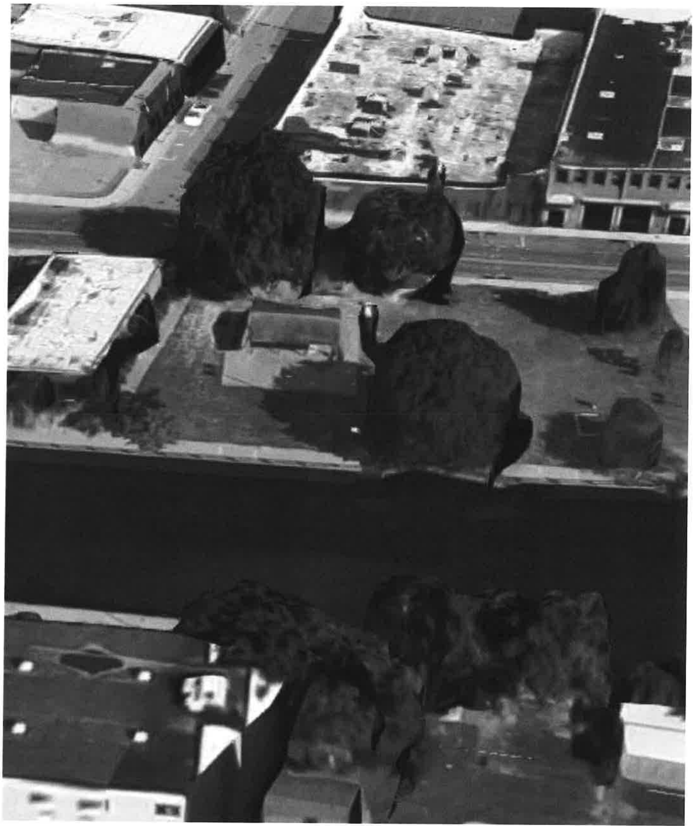
Aerial View (Rear Elevation)
