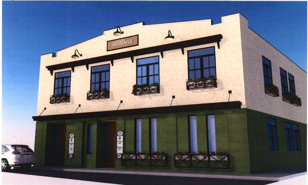
Side windows: Phase III
