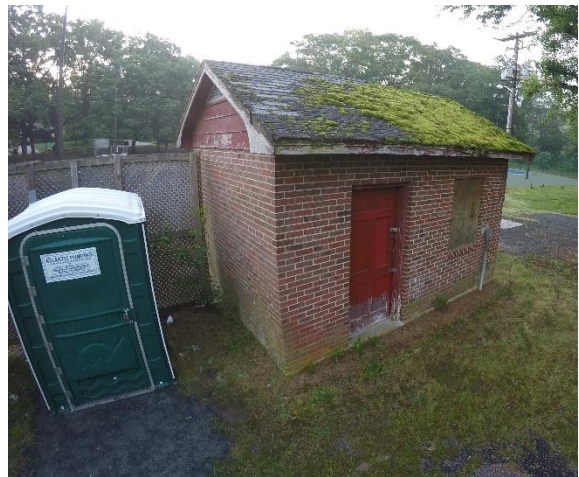
Potential Tennis Court Restroom
