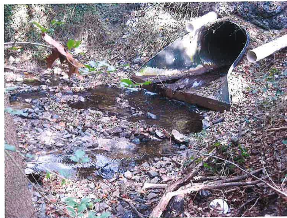
Stormwater Pipes discharging sediment & pollutants. Install Settling Basin to catch sediments and install Plants to remove pollutants prior to discharge into the Creek.
