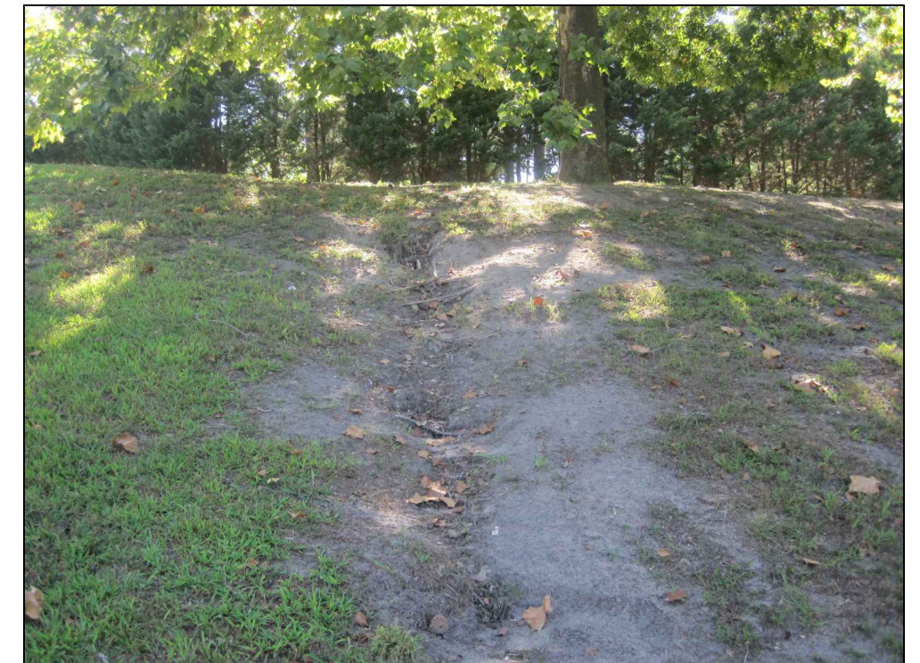
Unchecked erosion causing Sedimentation. Upgrade lawn areas by amending soils and selecting proper seed mix. Install biodegradable matting to stabilize soils. Begin yearly lawn maintenance / renovation at high-traffic areas. Convert lawn to native grass meadow where grades are too steep to maintain lawn.
