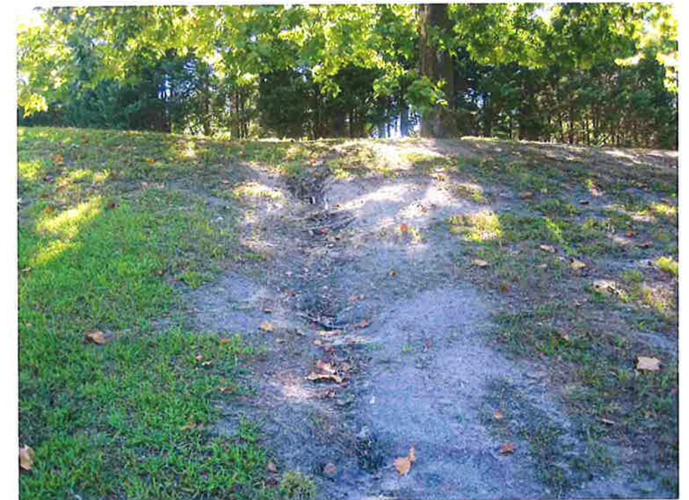
Unchecked erosion causing Sedimentation. Upgrade lawn areas by amending soils and selecting proper seed mix. Install biodegradable matting to stabilize soils. Begin yearly lawn maintenance / renovation at high-traffic areas. Convert lawn to native grass meadow where grades are too steep to maintain lawn.
