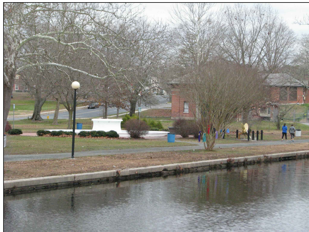
Channelization (concrete edge) Repair or replace with Natural Edge.
